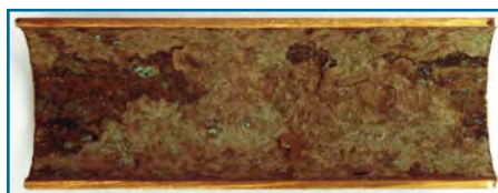
Figure 8. Microbiologically Influenced Corrosion (Source: Taprogge GmbH).
